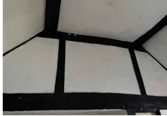
Detail of roof and ceiling cottage
